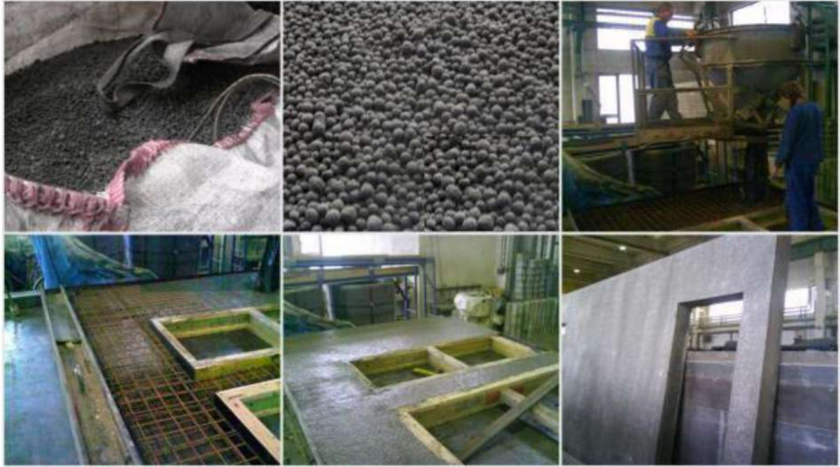
6 - Production of panels 20cm thick of lightweight self-compacting concrete with a density of (I.) 1750kg/m 3 containing LA
